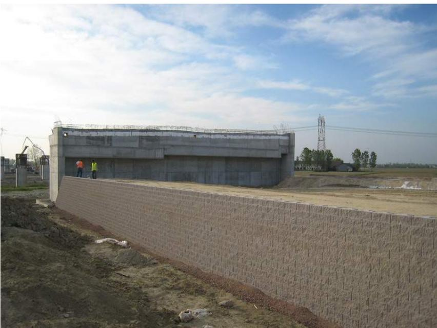
**Figure 11.** View of the segmental retaining wall
