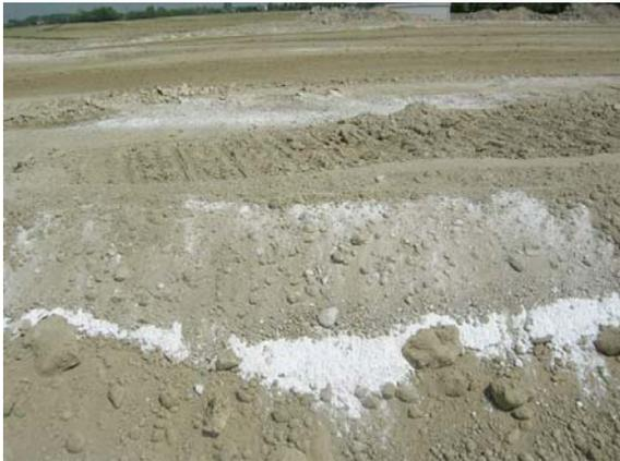
**Figure 4.** View of the lime stabilized soil
