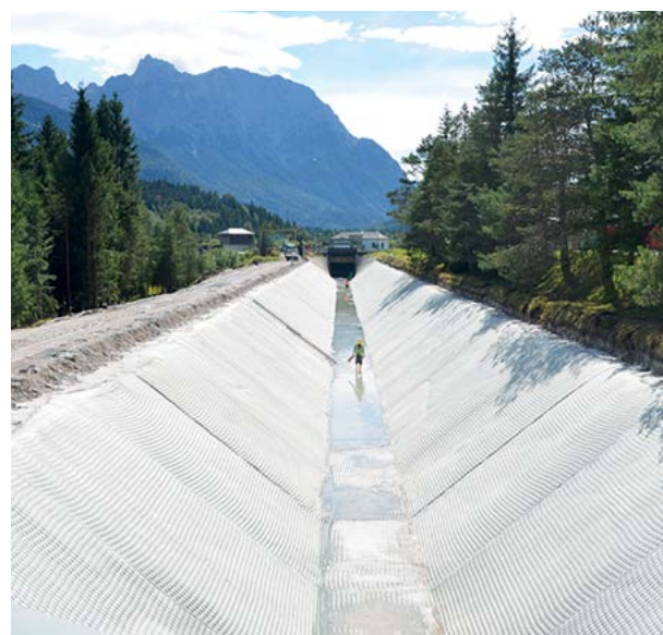
Canal refurbishment Germany, 2015, lining of Isar link canal using Incomat Standard geosynthetic concrete mattress.
