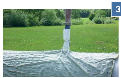
Concreting via filler neck
