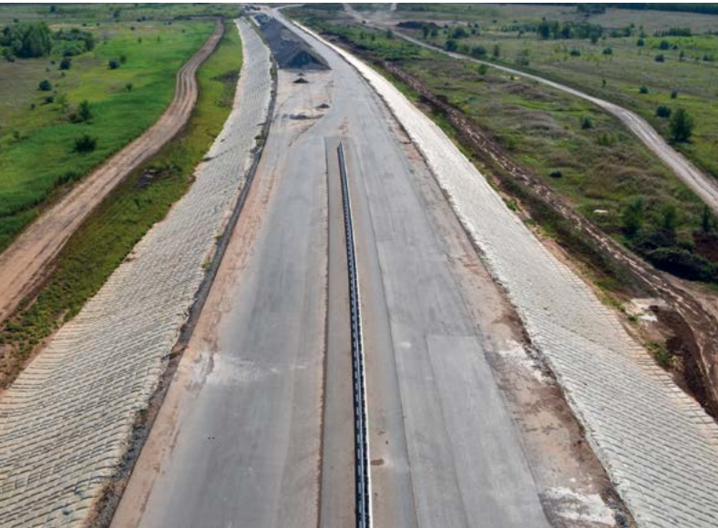
Embankment construction Russia, 2011 – 2014, protection of side faces of highway embankment slopes by Kirovsky bridge in Volga and Samara river floodplains using Incomat Flex.
