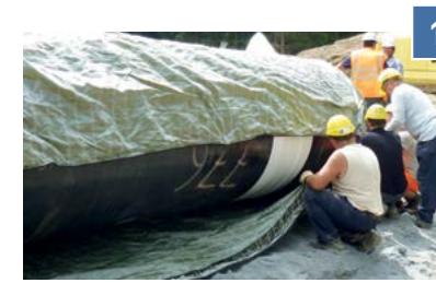
Fixing to pipe section
