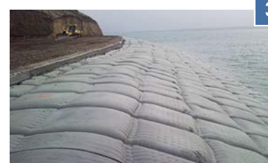
Filling of panels with fluid concrete/mortar
