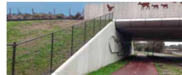
GRS Fortrac with prefabricated panels
