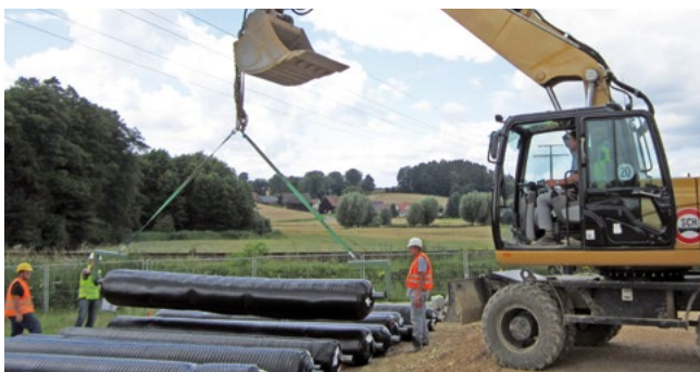
Use of lifting /laying gear
