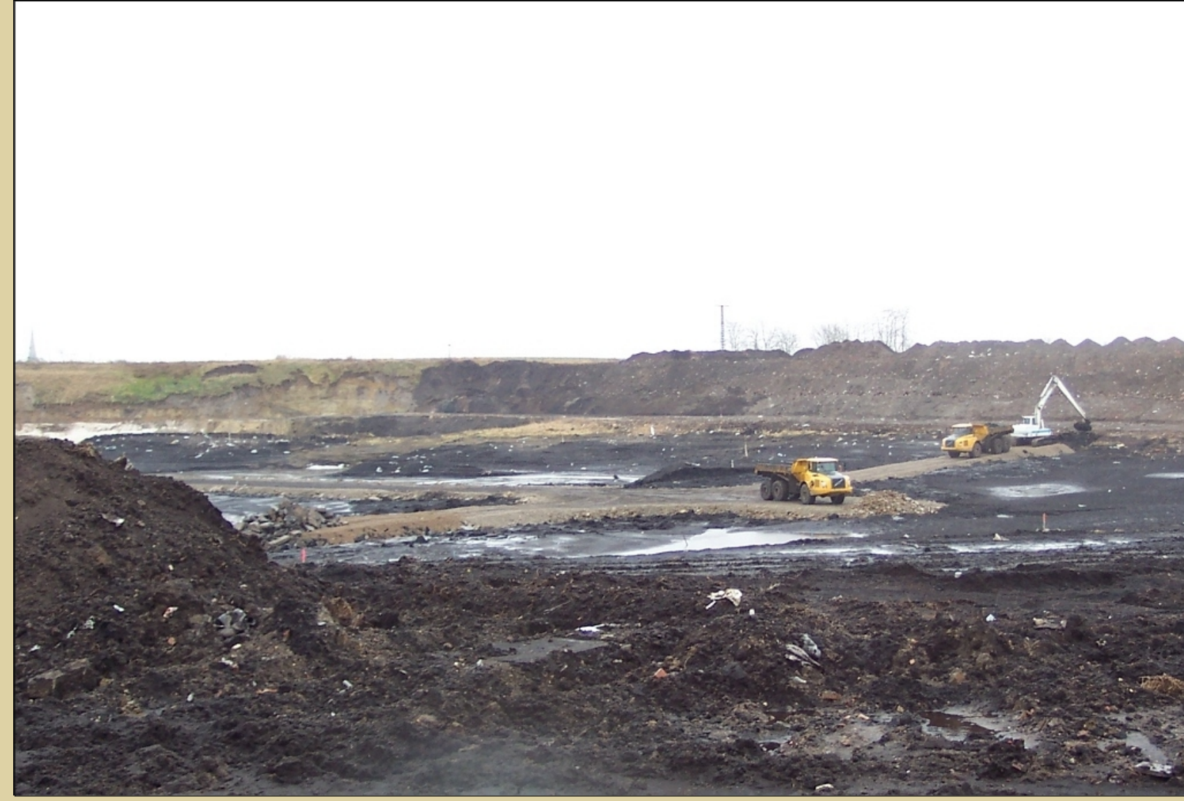
Construction of separation dams
