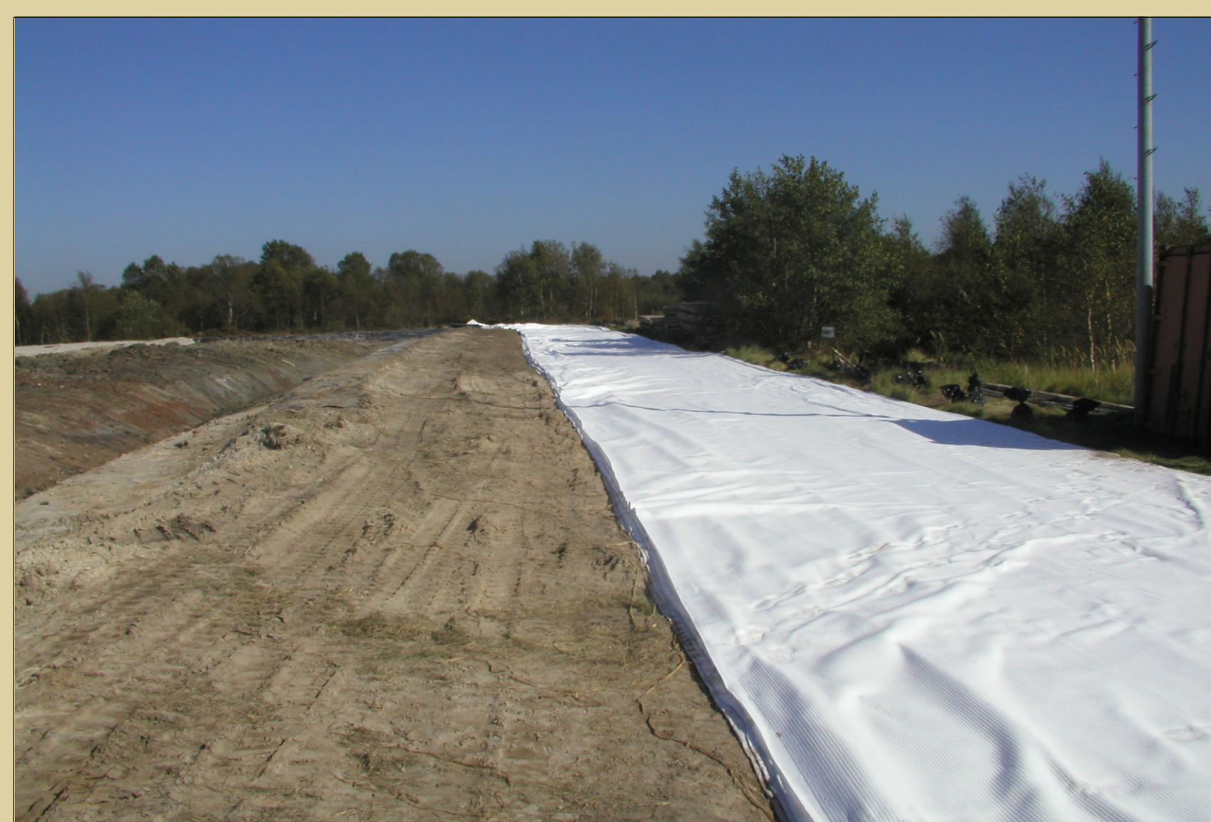
On site preparation of the panel
