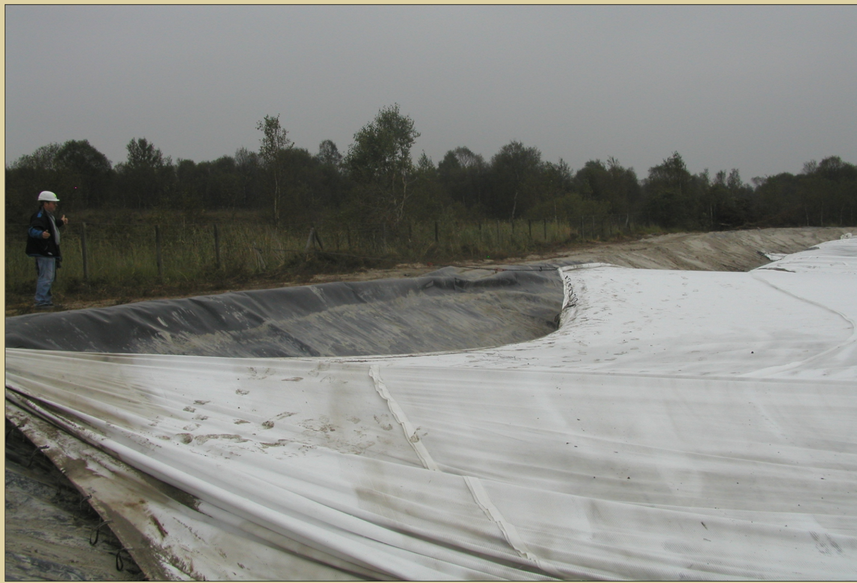
Installation of the panel
