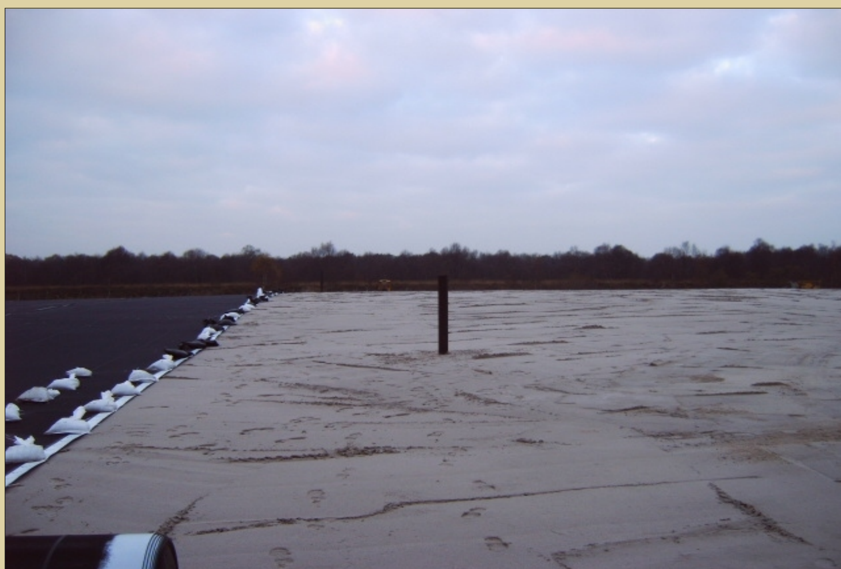
Installation of HDPE-membrane and geosynthetic drainage layer
