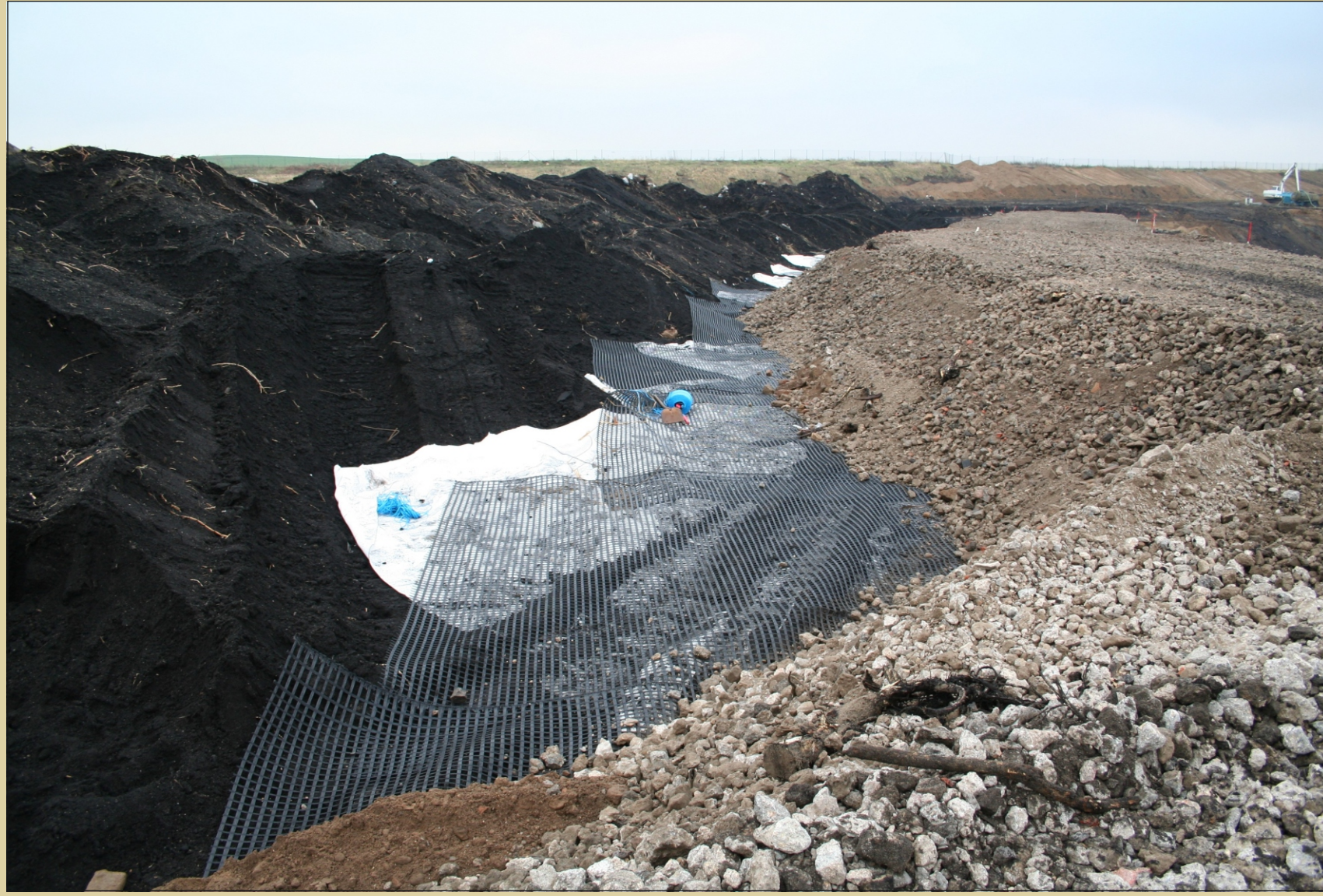
Anchoring of geogrids
