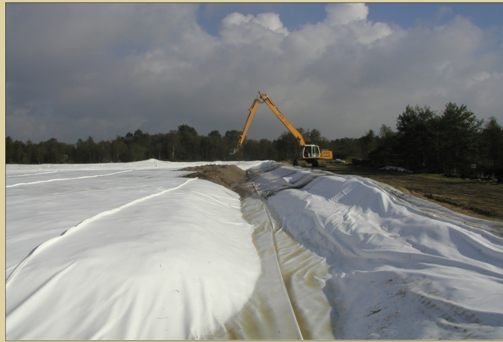
Filling the inner anchor trench
