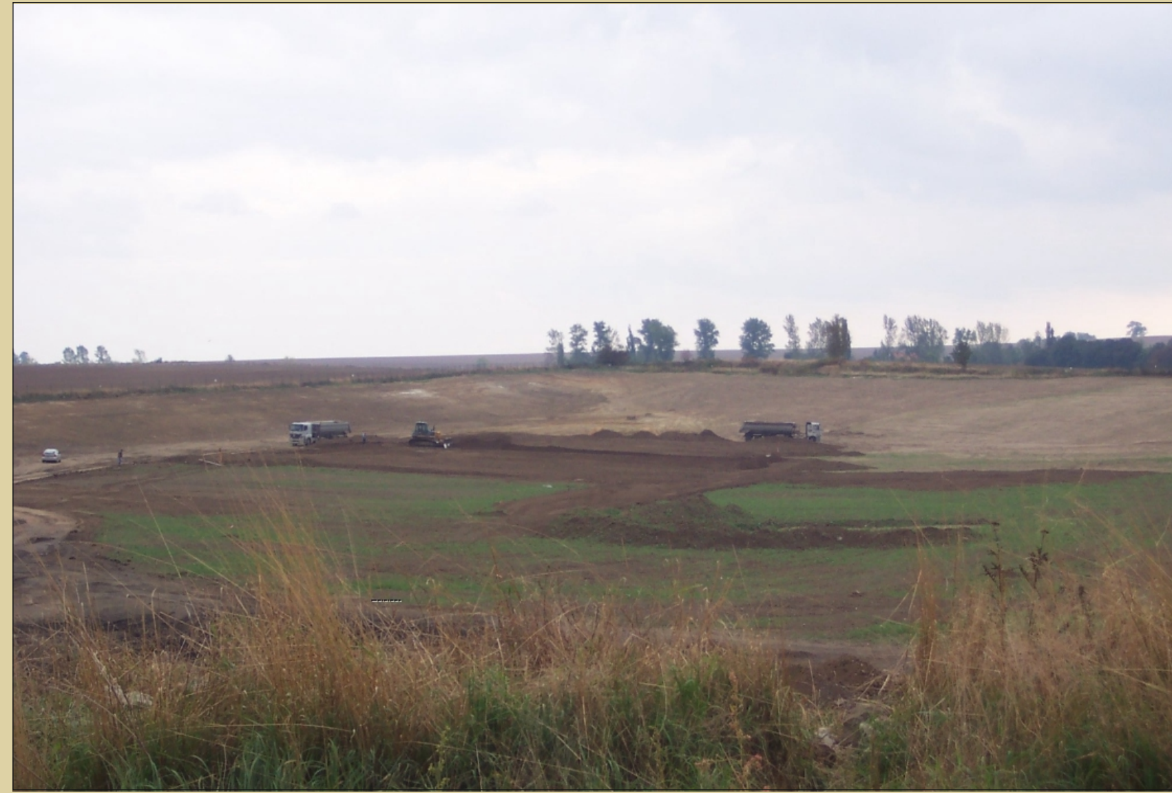
Profiling of final cover layer
