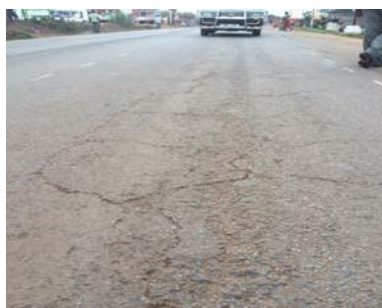
Figures 13a and 13b: Cracked existing surface
