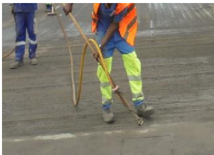
Figures 6a und 6b: Surface preparation after milling works
