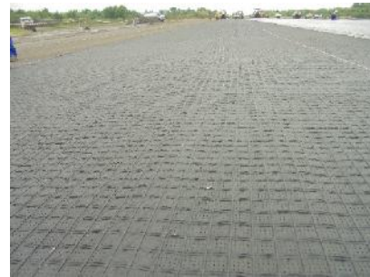
Figures 8a and 8b: Installation of PET Asphalt reinforcement grid
