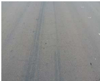
Figures 12a and 12b: Reflective cracks in a new rehabilitated road section after 5 months
