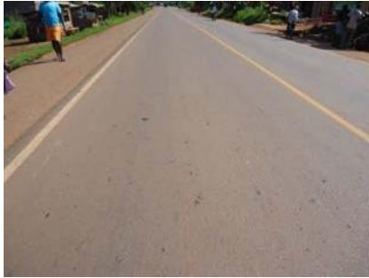
Figure 16a: Reinforced section after 1 year
