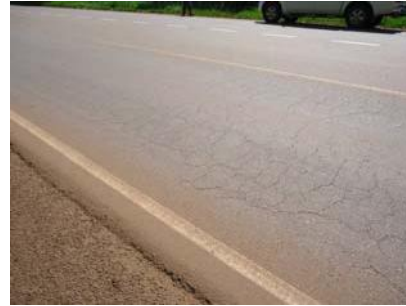
Figure 17: Unreinforced section after 1 year
