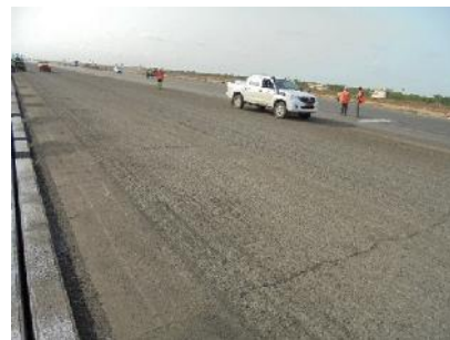
Figures 6a und 6b: Surface preparation after milling works
