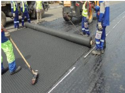
Figures 8a and 8b: Installation of PET Asphalt reinforcement grid
