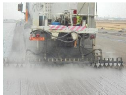
Figures 7a and 7b: Spraying of bitumen emulsion
