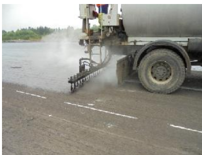
Figures 7a and 7b: Spraying of bitumen emulsion
