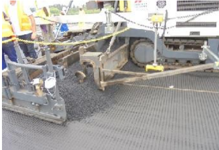
Figures 9a and 9b: Overlaying with asphalt incl. compaction
