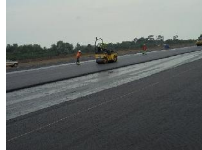
Figures 9a and 9b: Overlaying with asphalt incl. compaction
