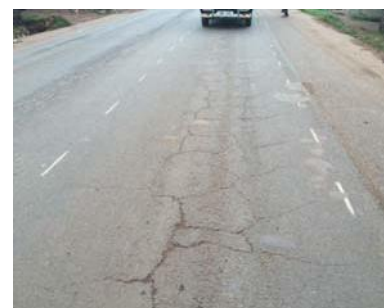
Figures 13a and 13b: Cracked existing surface
