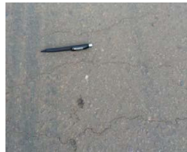
Figures 12a and 12b: Reflective cracks in a new rehabilitated road section after 5 months
