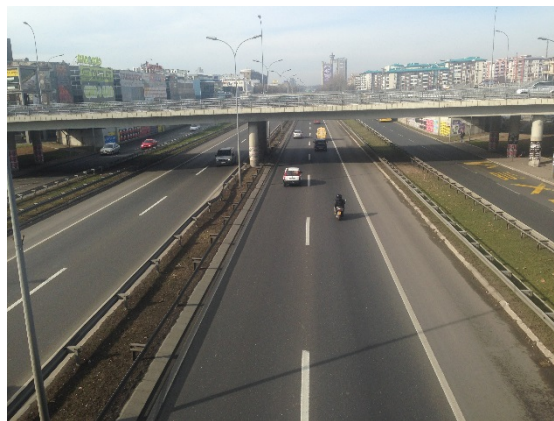
Figure 10. E75 pavement condition in 2016
