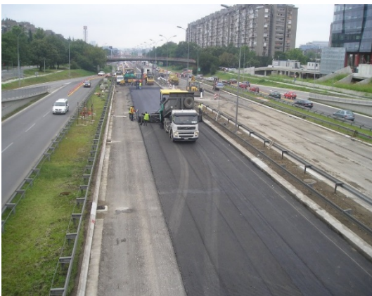
Figure 9. Asphalt placement on HaTelit
