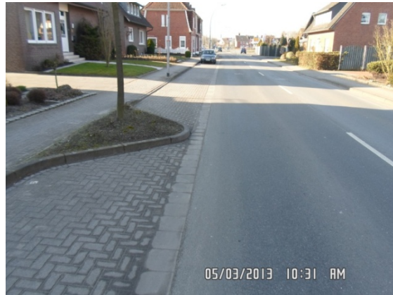
Figure 5. Condition in March 2013
