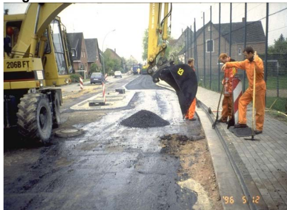
Figure 7. Repair works at the road edge in 1996
