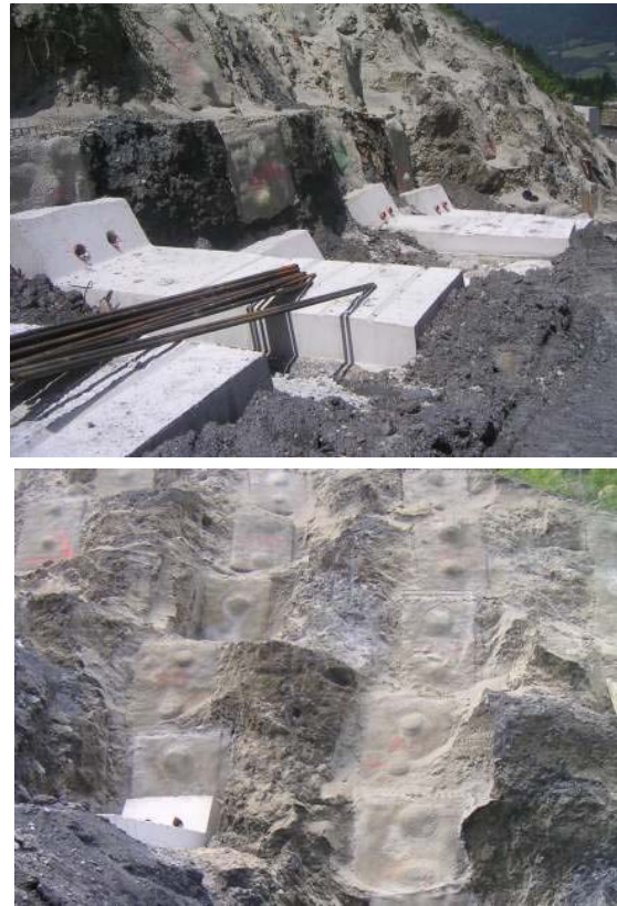
Fig. 10 Measures to stabilize and drain slope cuttings at foundation level
