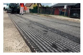
Viewed in the driving direction of the asphalt paver the end of a layer always covers the beginning of the next layer to prevent it from being lifted. If several lanes are place side by side or behind each other, overlaps shall be arranged with offsets to prevent multiple overlaps occurring at the same location.
