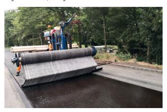
At structures such as gully holes or manhole covers SamiGrid can be simply cut out with a knife.
