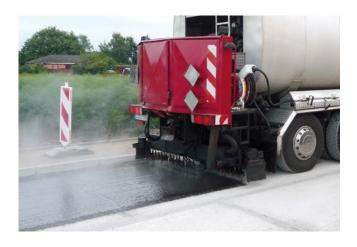
When installing SamiGrid on a milled concrete surface, it is recommended to spray an initial 200 – 300 g/m² of the bitumen emulsion as a dust control measure.
