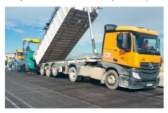
Paver and transport vehicles must be moved carefully and cautiously to keep the shear stress on the composite as low as possible.
