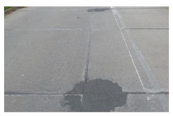
Individual cracks with a width of less than 3 mm may remain untreated. Expansion joints and cracks wider than 3 mm should be filled with a bituminous sealant after cleaning.
