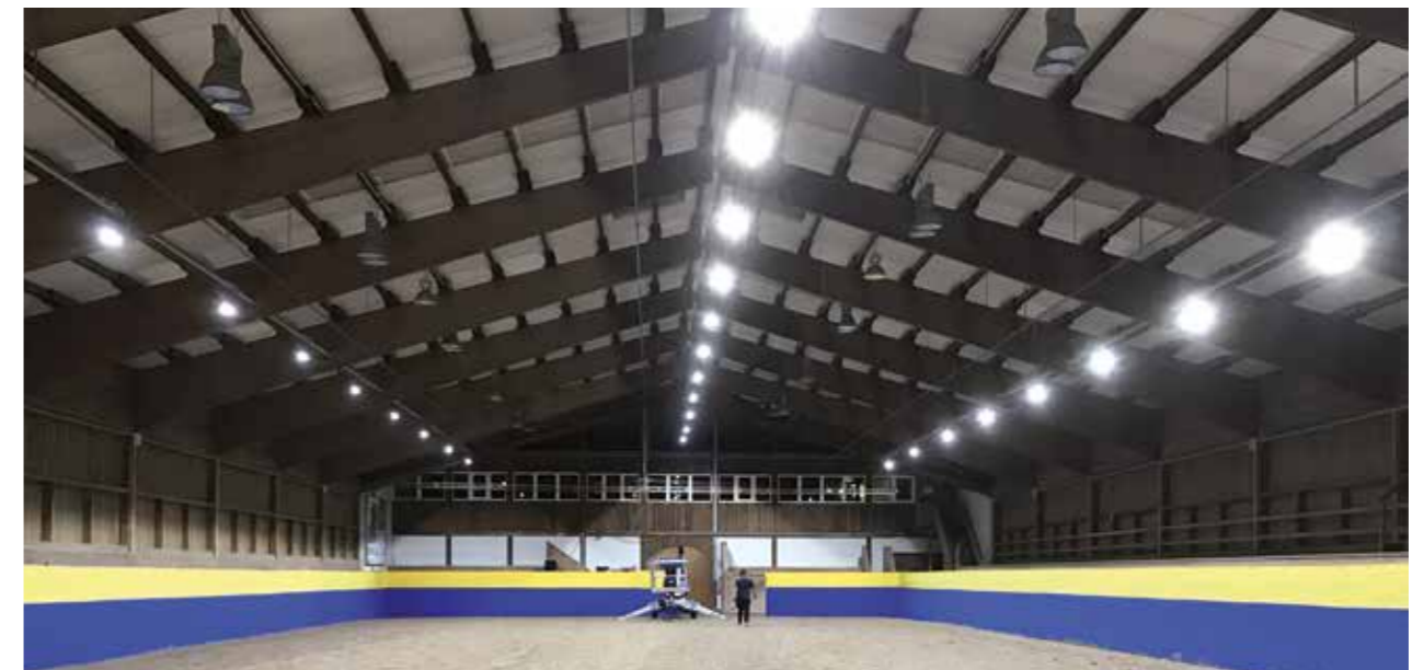
Optimal training and tournament conditions through the use of Lubratec LED luminaires.
