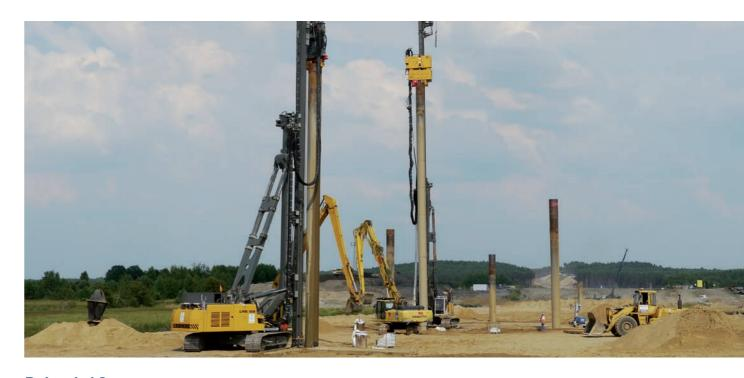
**Poland, A2 motorway** Poland, 2010 – 2011, construction of embankment with 3,400 Ringtrac columns for A2 motorway near Jordanowo. With a length exceeding 30 m, these were the longest geotextile-encased columns installed to date.
