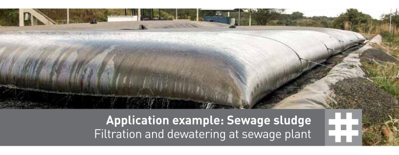
A bioreactor at the ETE Uberabinha sewage plant in Brazil produces waste water containing organic particles in suspension. The particles had previously been removed by means of a flotation process, with the floated sludge being returned to the bioreactor. However, the chemicals used in this method slowed down the reaction process.
