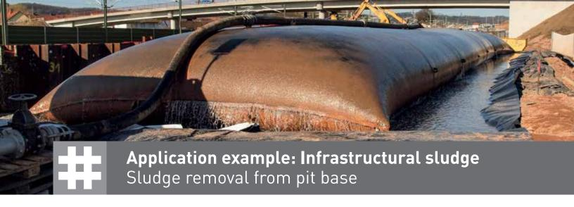
An excavation pit in Neuhof in the German Federal State of Hesse contained a 3 ft (1 m) layer of sludge topped by 13 ft (4 m) of water. The sludge had to be pumped off to allow the pouring of an underwater concrete foundation. For excavation stability reasons, casting had to take place prior to removal of the water.
