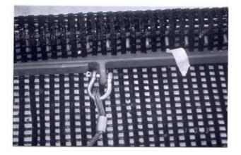
Figure 3. Tension bar used to tighten the aramid geogrid during installation
