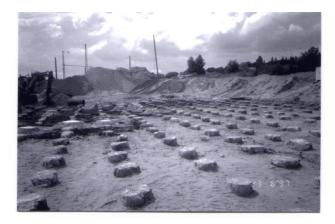
Figure 8. Project Rathenow (,Körgraben') : cemented stone columns before installation of aramid geogrids
