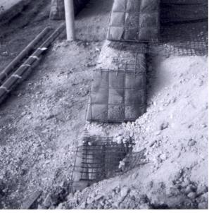
Figure 13. Unterkaka Logistics Centre: construction stage, PVA-geogrids, GeoGreen<sup>R</sup>-gabions, connections, fill soil
