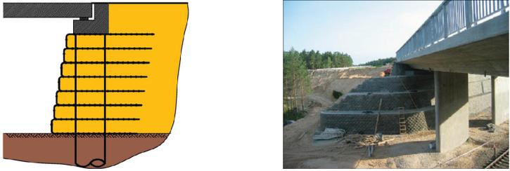
Figure 1. GRS as front and wing wall facing of bridge abutments (not loaded by the sill beam).
